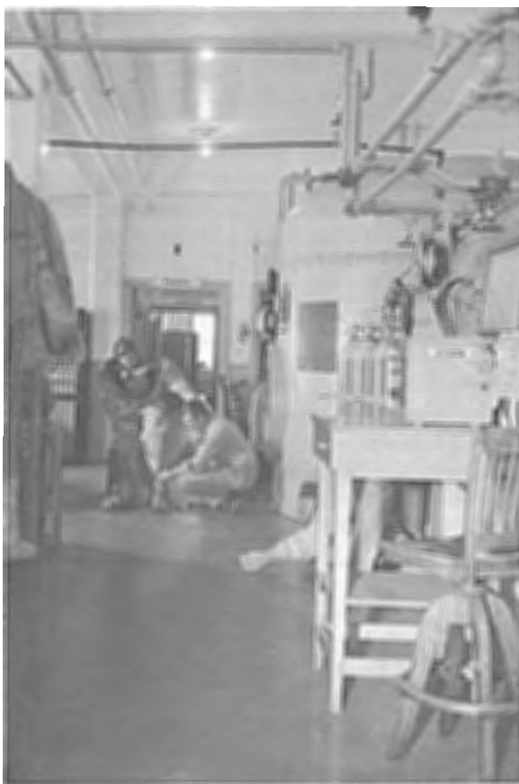
FIGURE 1-4.—“Igloo” and recompression chamber, Deep Sea Diving School. Above each pressure tank is an access chamber (igloo), and a recompression chamber (right) is connected to the igloo.
