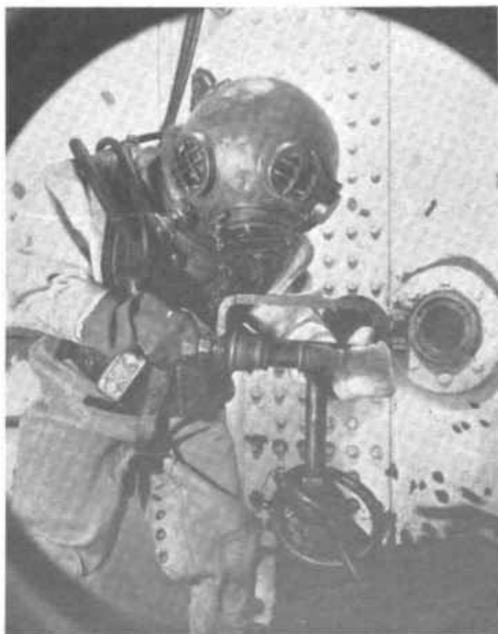
PLATE 2—FIGURE 2.—Diver in water diving tank sawing through a section of steel piping.
