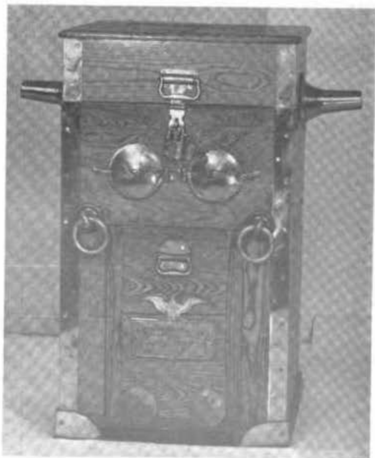
PLATE 55.—Navy standard diving air pump, Mark III, assembled— Front view.
