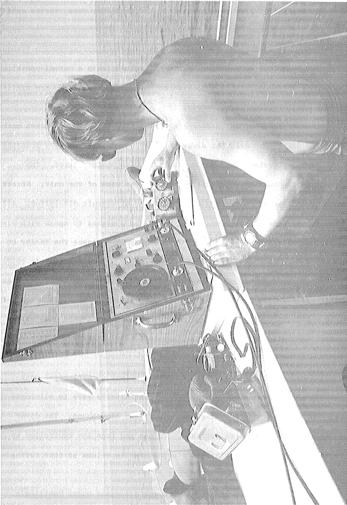
FIGURE 5-7. Hardwire communications system and stop watches for timing dives (Photo by author).
