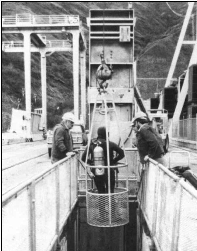
FIGURE 12.15 Line-Tended Diver Lowered into Dam Gatewell
