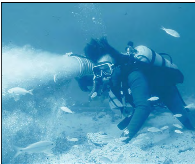
FIGURE 9.45 Backfilling with an Injection Dredge
