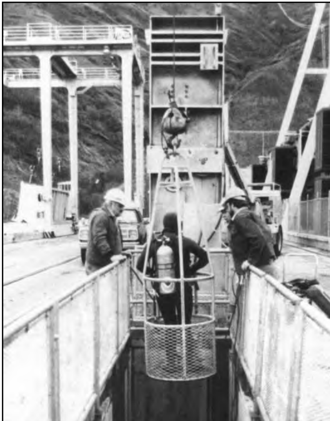
FIGURE 12.15 Line-Tended Diver Lowered into Dam Gatewell
