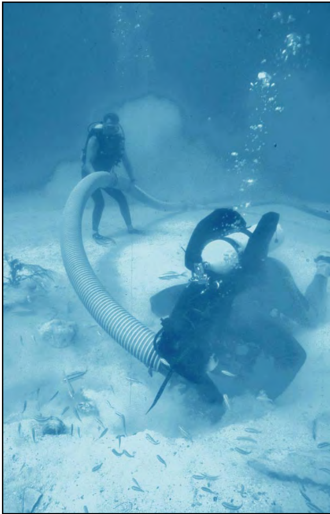
FIGURE 9.44 Excavating with Injection Dredge
