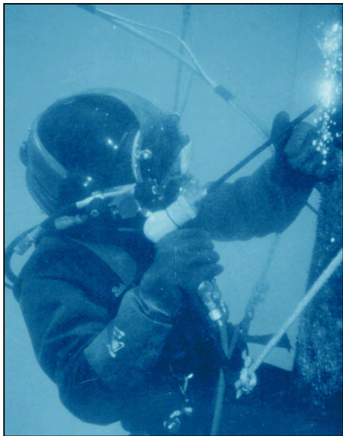
FIGURE 10.16 Ultrathermic Oxy-Arc Process
