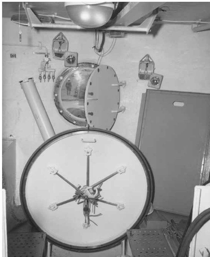
Fig 5. SEALAB II Main entry hatch open. Note tile shower to left, diagonal stuffing tube, 4 emergency air hose bibs, 2 emergency lanterns, and humidity sensor in ceiling. (Official photograph, U.S. Navy)
